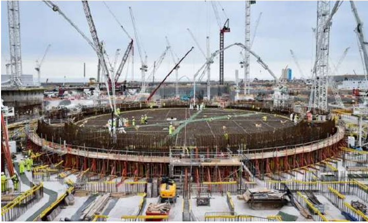
The base of the first reactor at Hinkley Point C is prepared for the UK's biggest ever concrete pour. Photograph: Ben Birchall/PA
